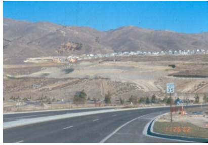
INITIAL CUT AND FILL SLOPES 11/2002
